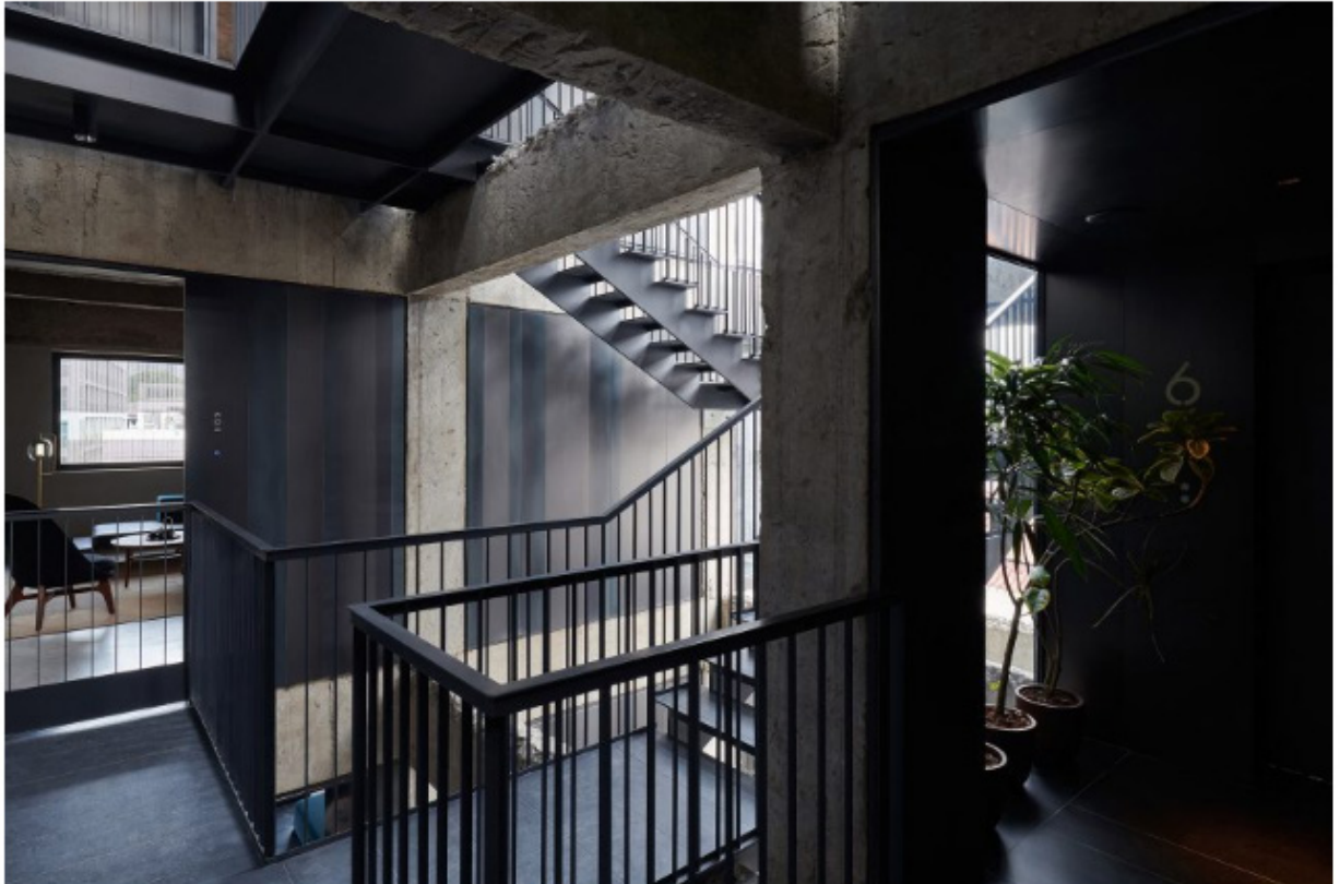
Neri&Hu inserted a new metal stairwell into the old structure
