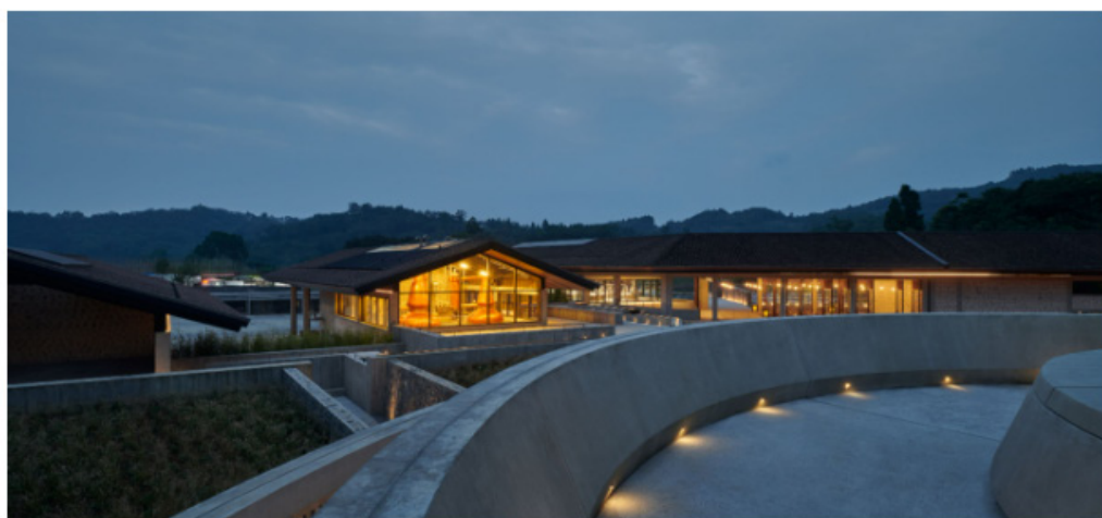
THE ROOFS OF THE THREE WHISKY PRODUCTION FACILITIES USE RECLAIMED CLAY TILES AND THE INFILL OF ROCK WALLS IS MADE FROM THE VERY BOULDERS EXTRACTED FROM THE GROUND DURING SITE LEVELLING
