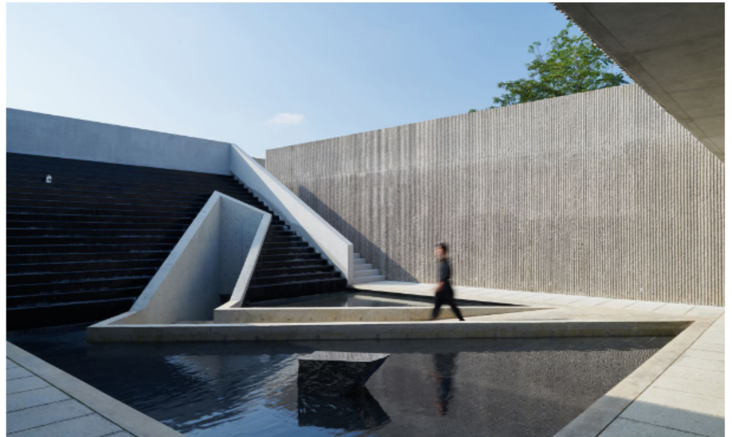
THE SQUARE BUILDING HOUSES A RESTAURANT AND BAR OVERLOOKING A COURTYARD OF WATER THAT IS DESIGNED AS AN ENGAGING FEATURE.
